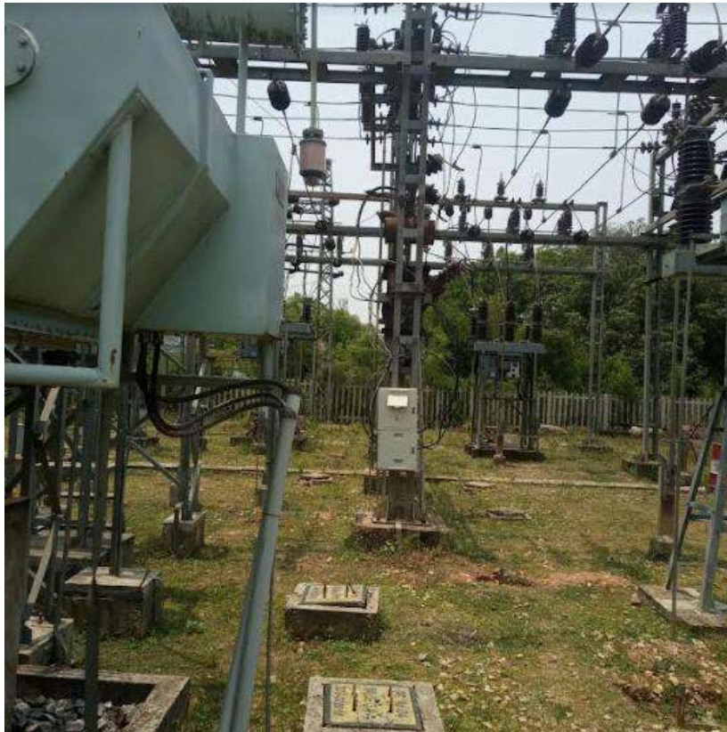
Visit to 33/11 kV Betanati substation
