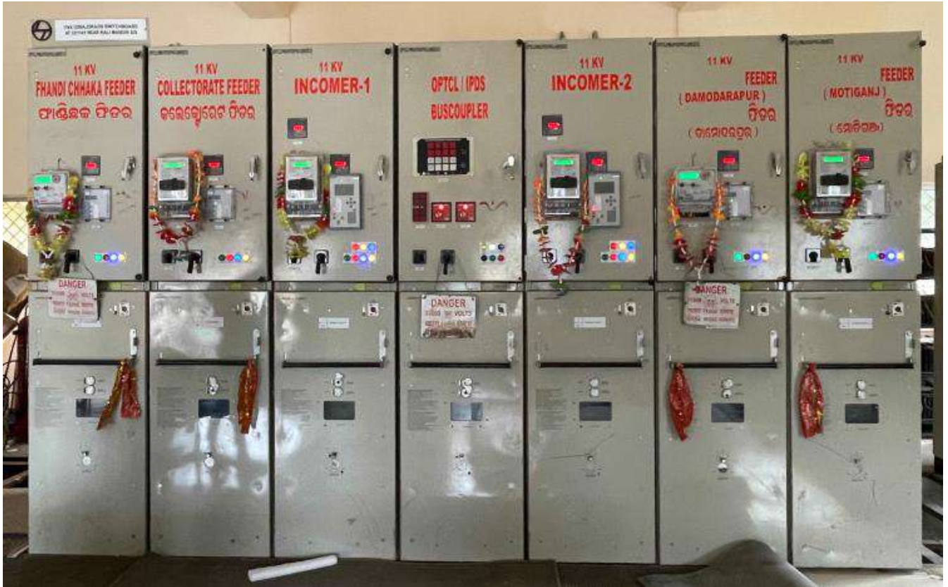
Control Panels at the 33/11 kV Kali Mandir Sub-Station
