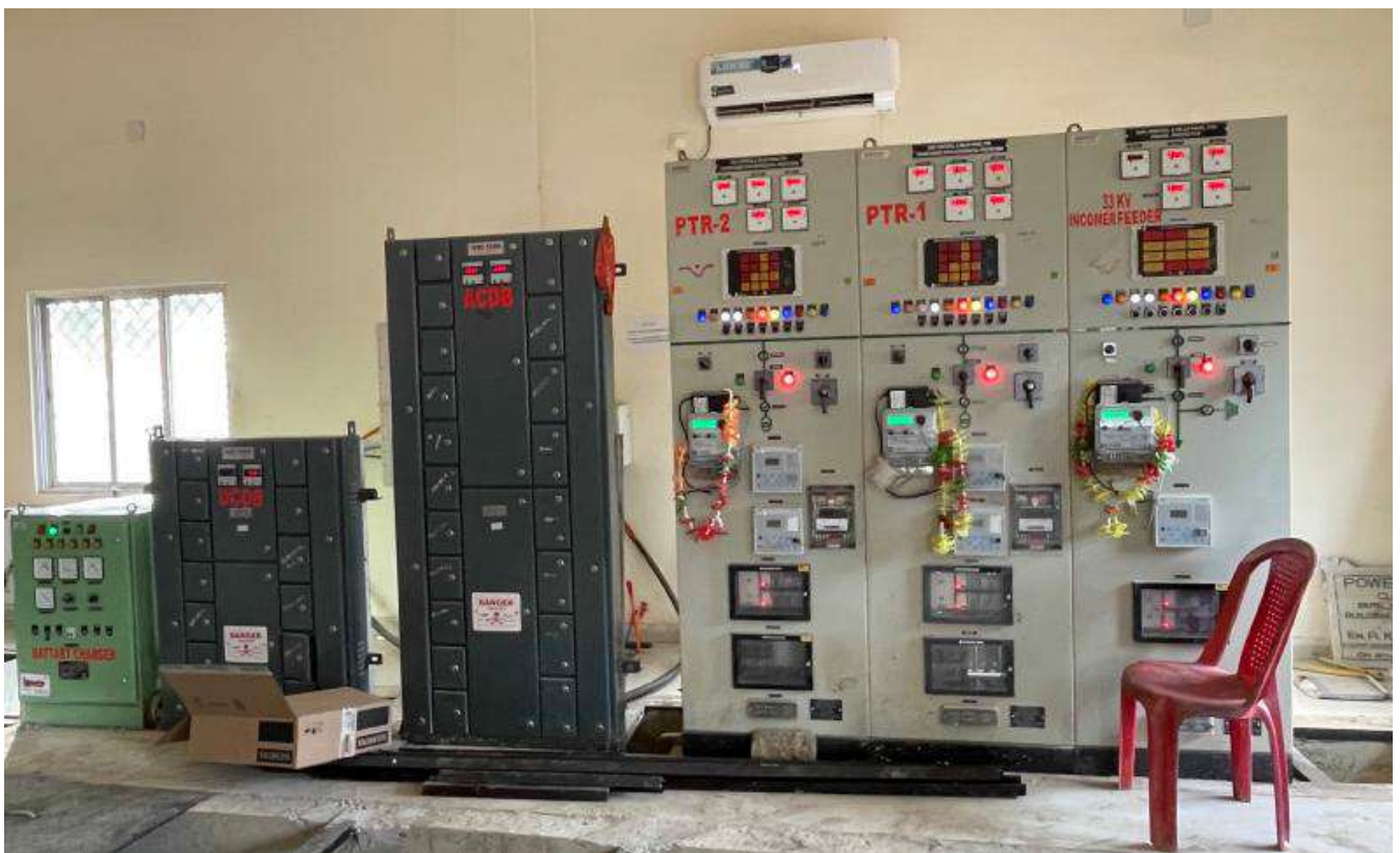
Control Panels at the 33/11 kV Kali Mandir Sub-Station
