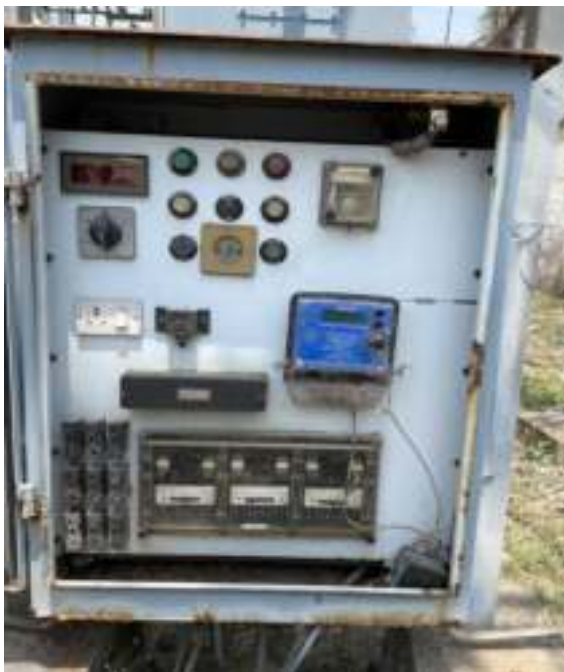
11 kV and 33 kV Control Panels at Ganeswarpur 33/11 kV PSS.
